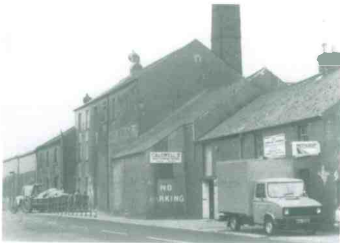
Restructuring and sub-division of older Industrial premises is required
