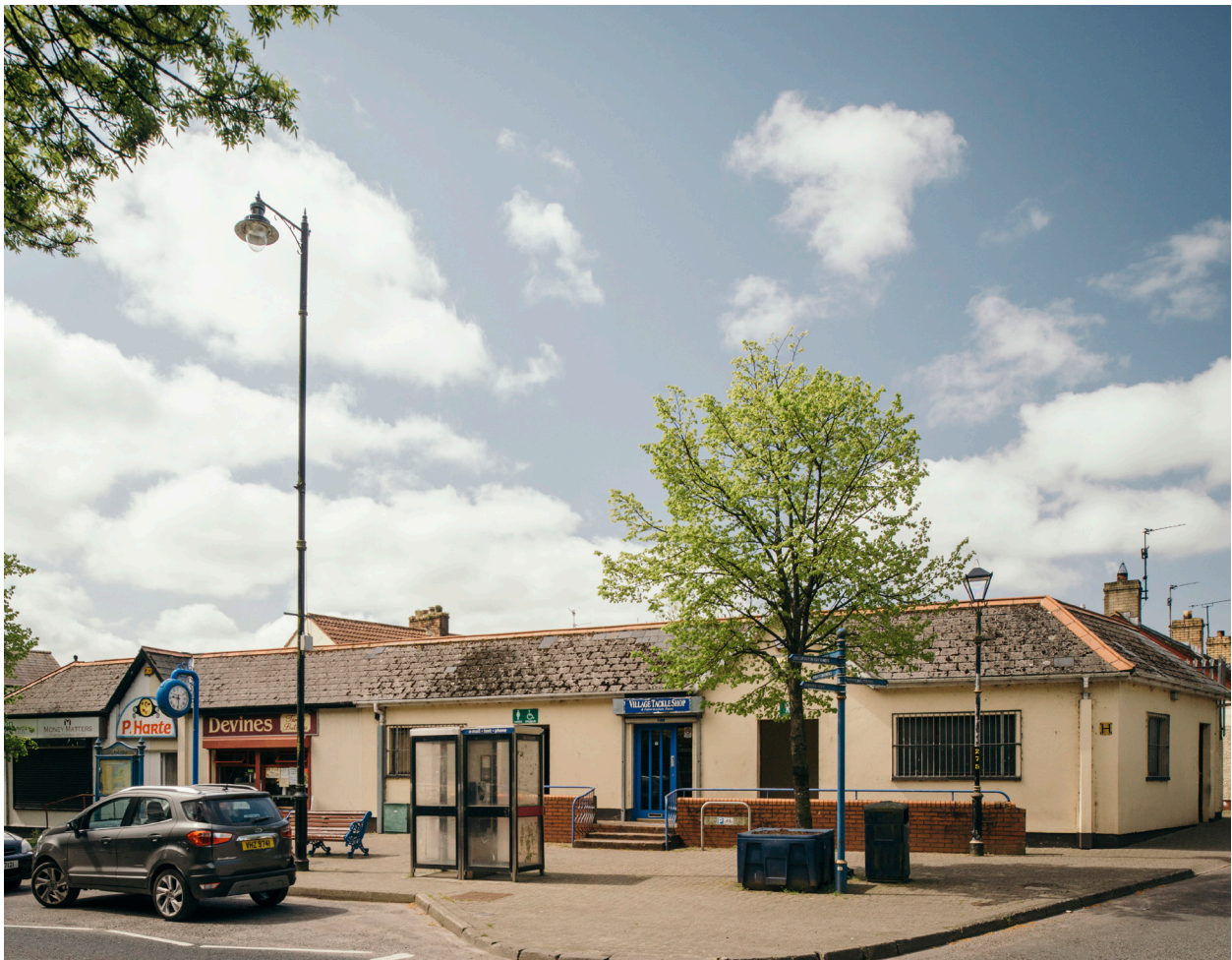
The existing public toilets - a potential refurbishment opportunity to provide more / higher quality retail units
