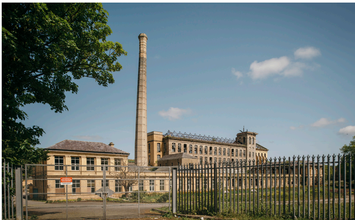
The Herdman's Mill complex ceased spinning linen in 2004. A subsequent change in ownership has failed to find viable, contemporary uses, leaving this major heritage asset vacant, physically deteriorating and vulnerable to arsonists.
