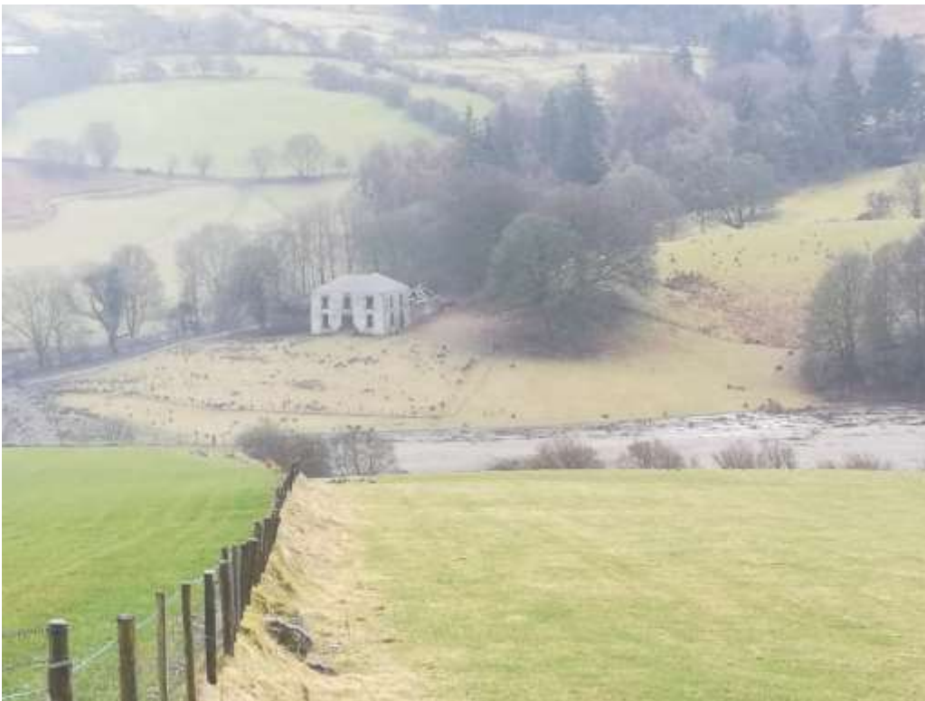
Derelict vernacular property alongside the Glenelly River
