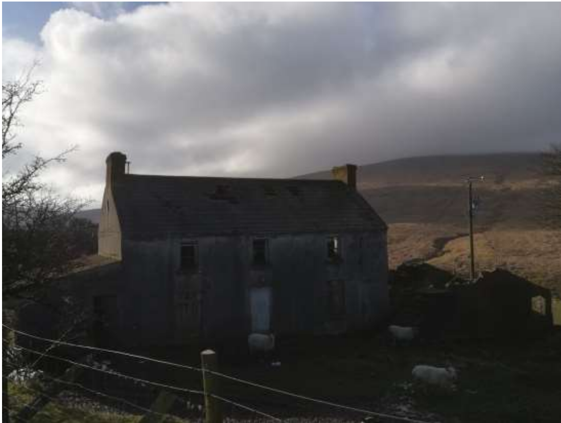
Derelict vernacular farmhouse near Sawel & Dart.
