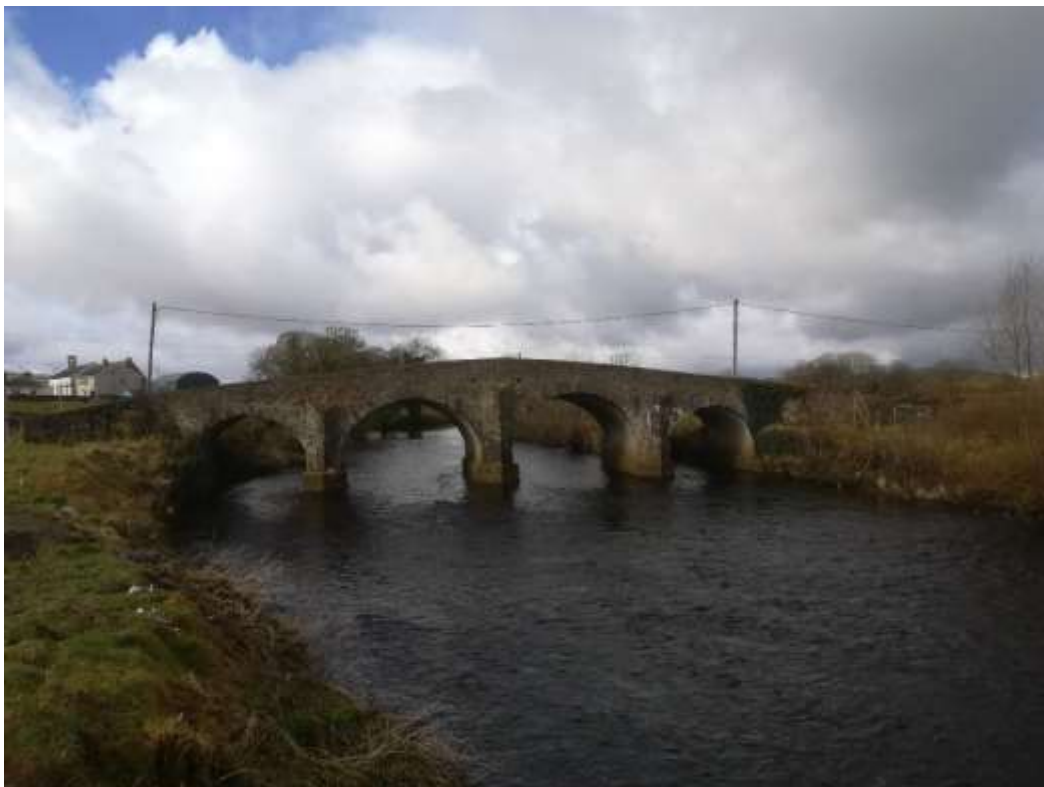
Multi arched stone bridge at Killeter.
