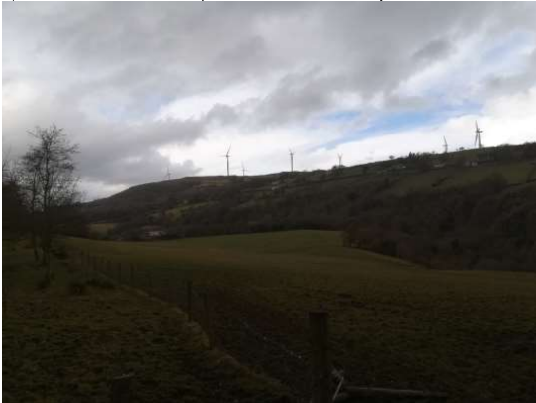
Slievekirk Windfarm on the northern side of Bonds Glen.
