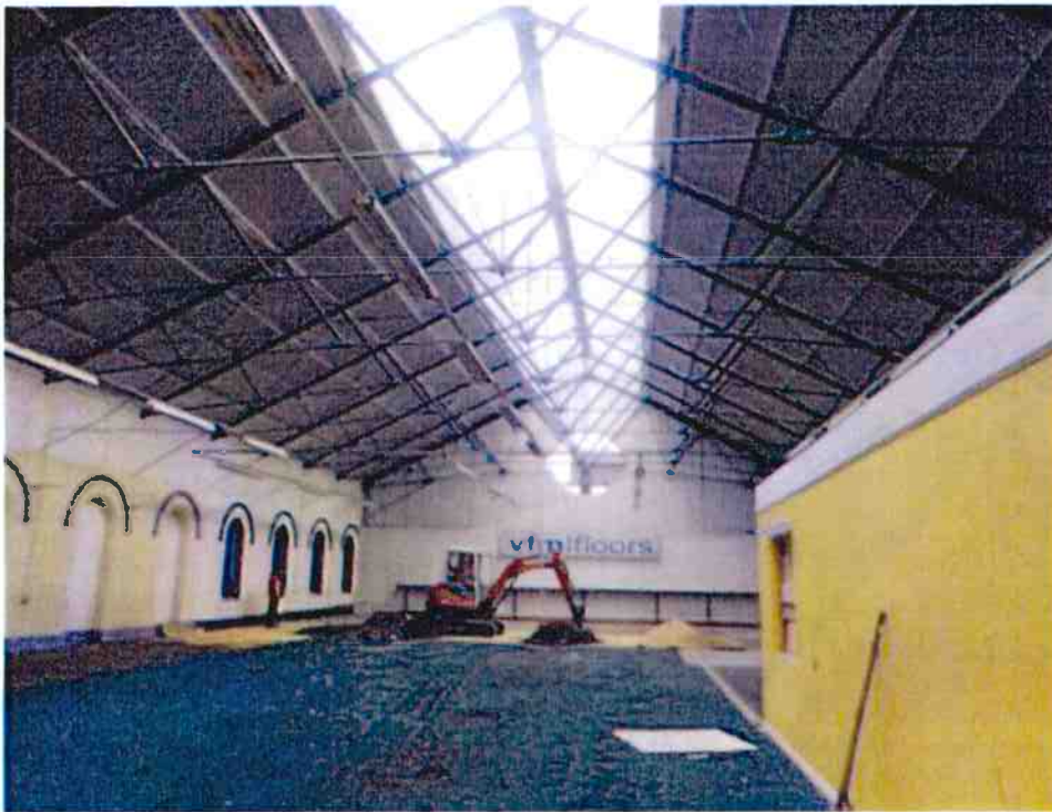
Photograph 12 Interior of Former Siding buildings
