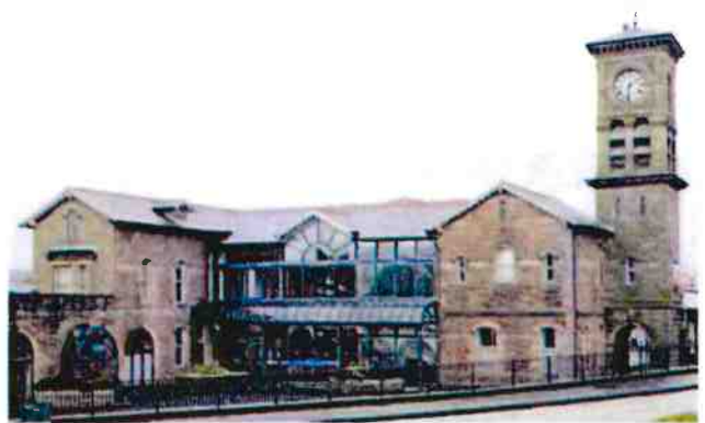
Station with existing new section to centre
