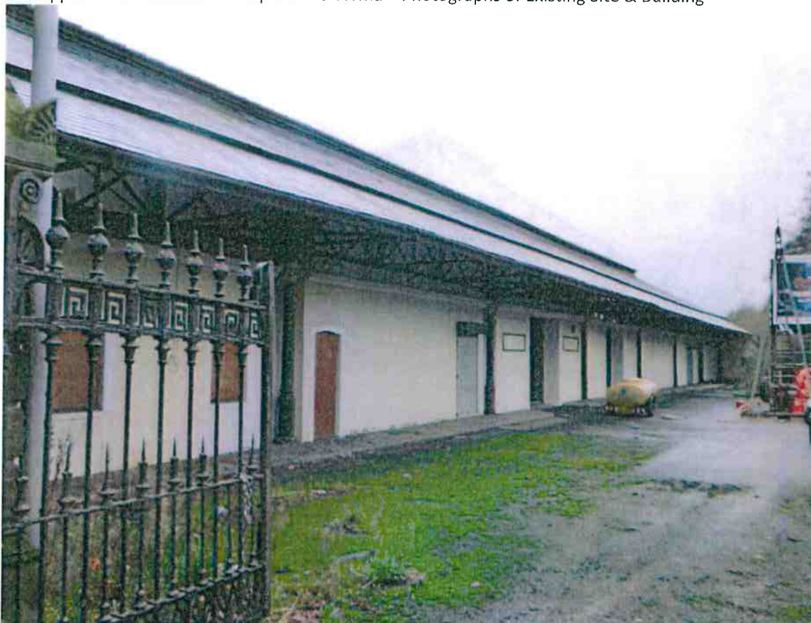
East Elevation – Block infill to former open sided Railway Shed
