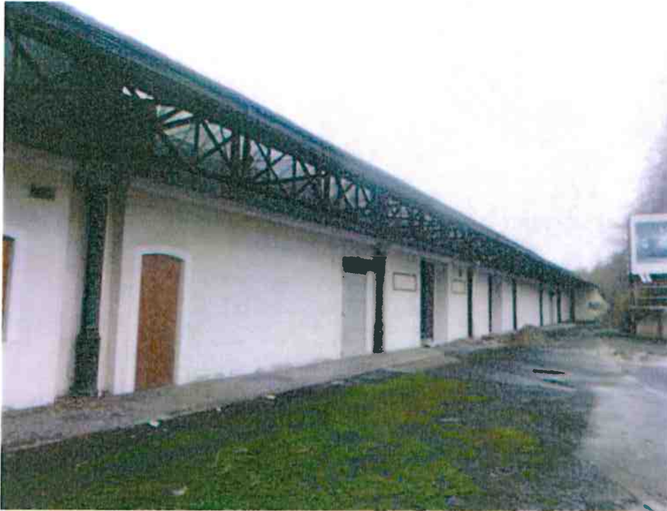
Photograph -9 Former railway buildings with open roof structure
