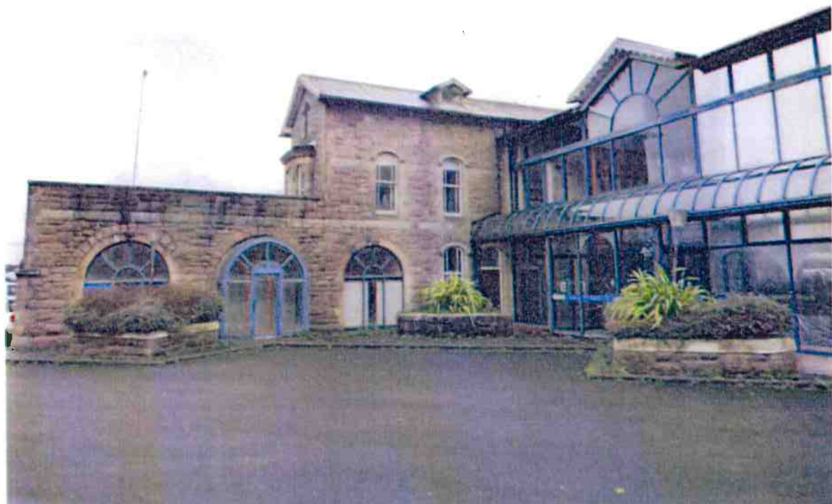
Remaining South west wing and modern infill
