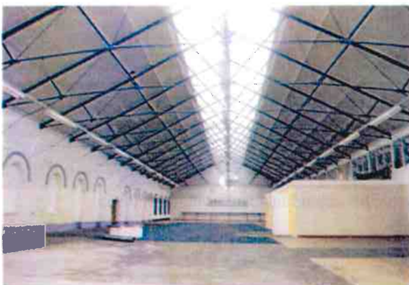
Current Interior of Former Railway Shed
