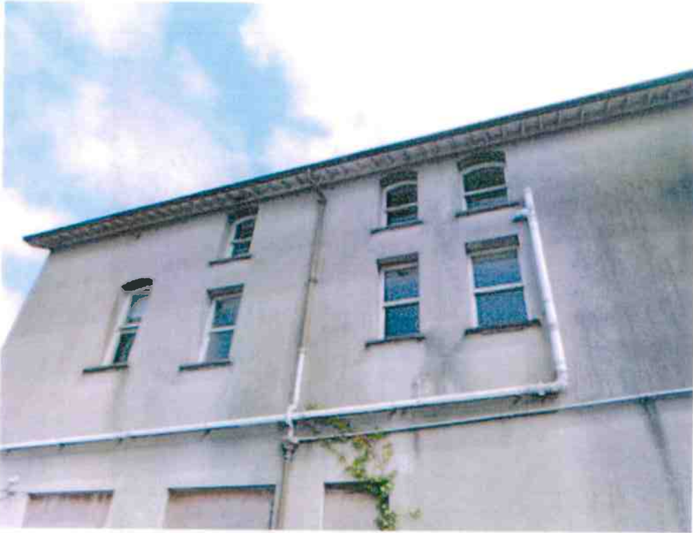
Photograph 5 Building exteriors to west of tower
