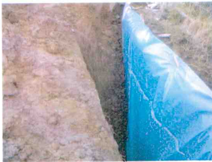
Examples of vertical root barrier techniques
