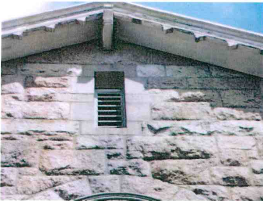
Photograph 14 Roof detail of tower
