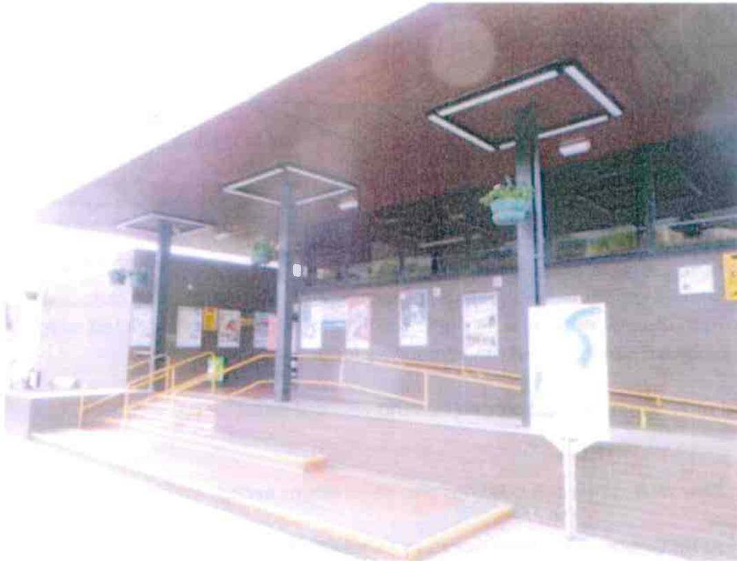
Photograph 17 Existing Rail Station
