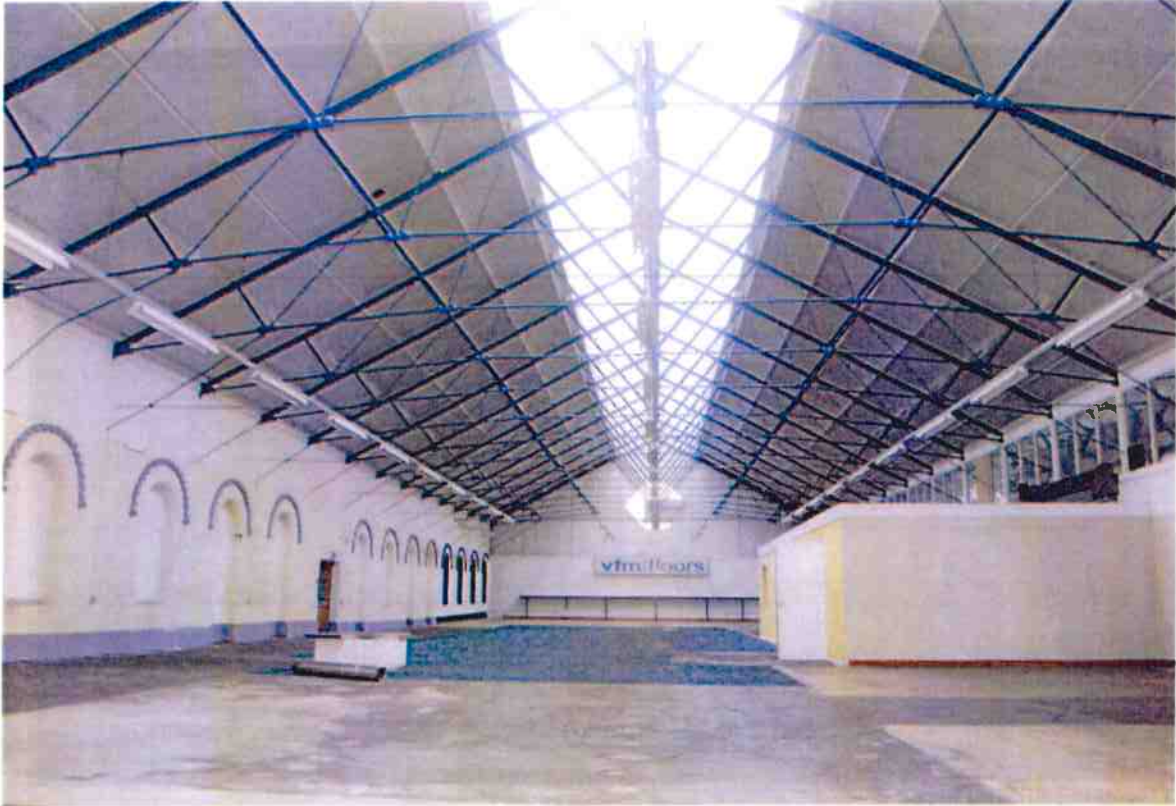
Interior of Railway Shed
