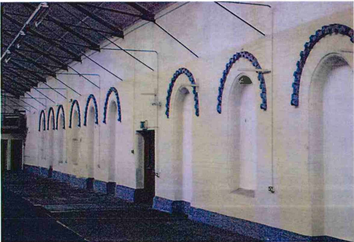
Former openings to side of shed
