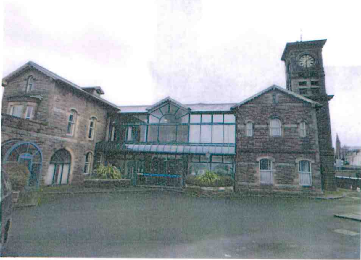
Front View to South Elevation with modern infill
