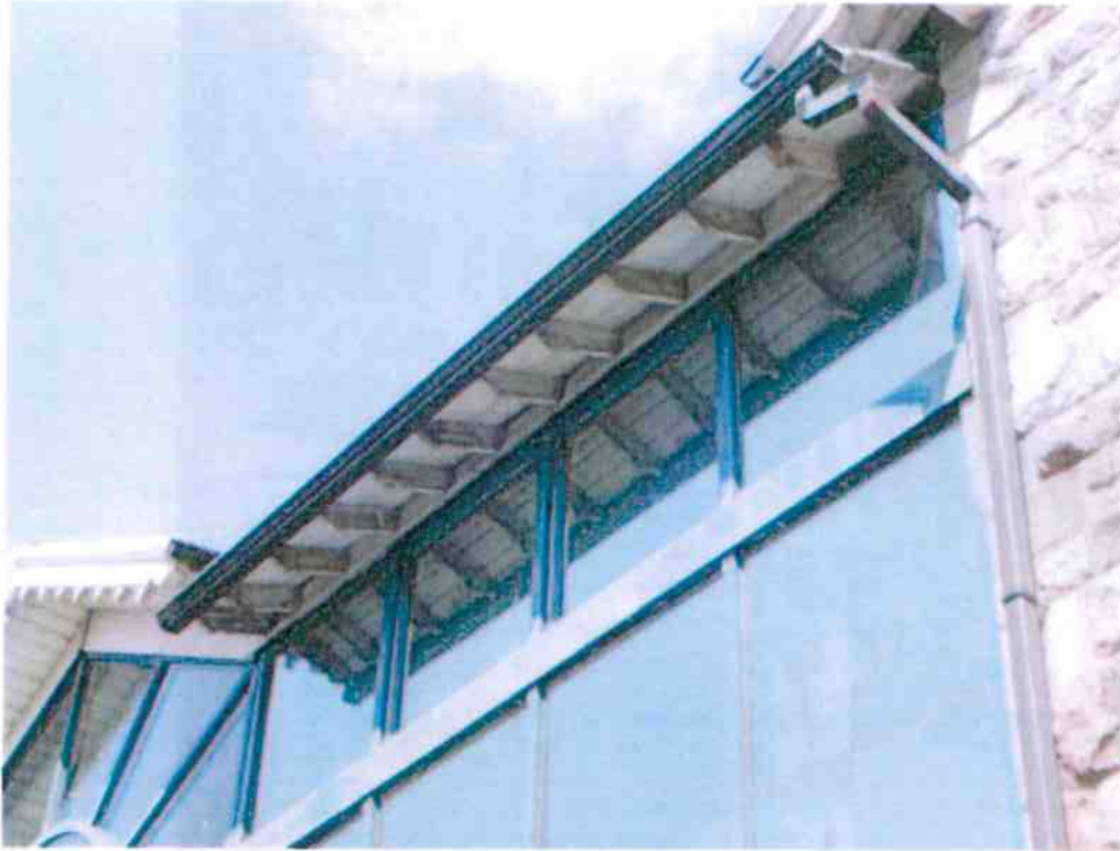
Photograph 13 – Roof detail of modern building connection
