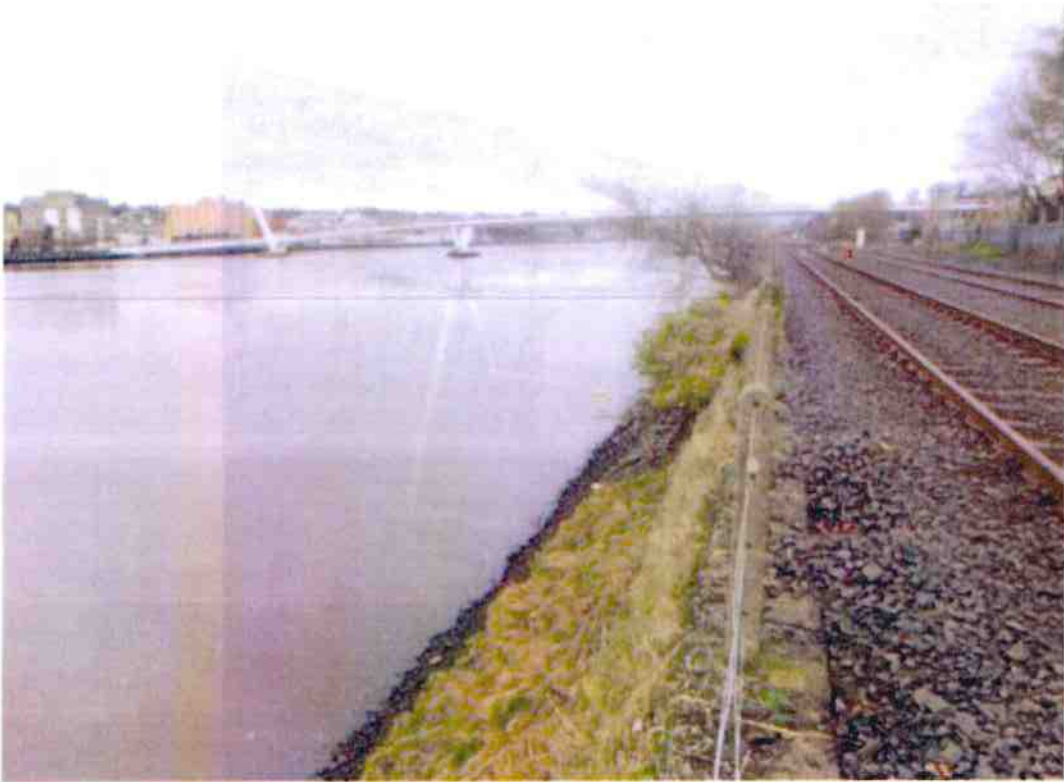
Photograph 7– Railline and edge with River Foyle.
