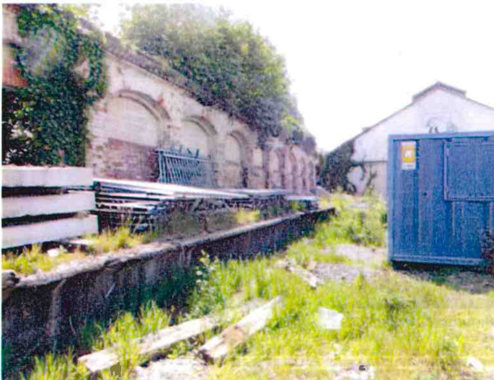
Photograph 16 Former platforms and gable end of former siding buildings
