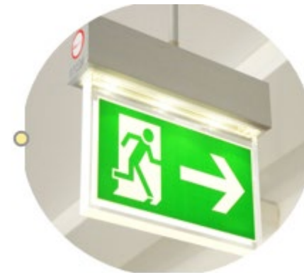
Emergency Lighting Cert.
