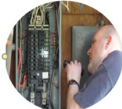
Electrical Inspection Cert.
