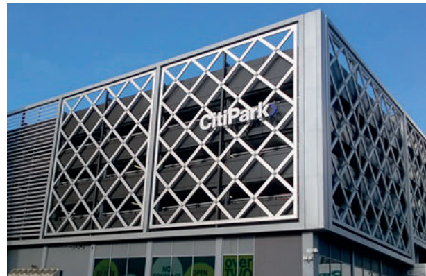
High quality multi-storey carpark, Nottingham
