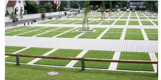
Sustainable Urban Drainage System car parking
