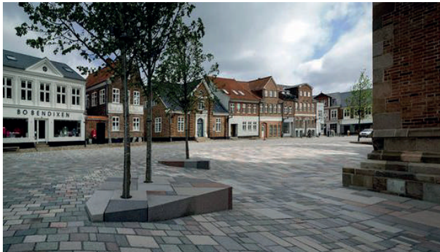
High quality public realm works
