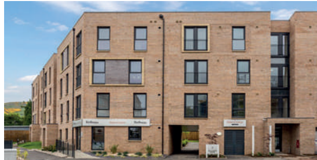
Residential development of a sustainable density that adds to placemaking of the site should be encouraged, Edinburgh
