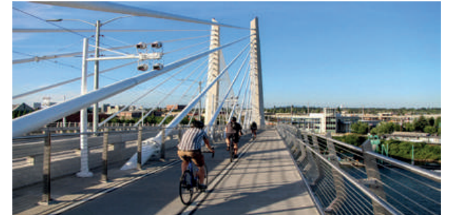
Bridge with cycle capacity, Portland Oregon
